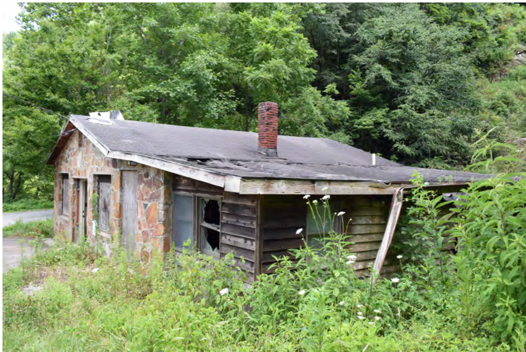
West elevation of the store, view to the east-southeast
