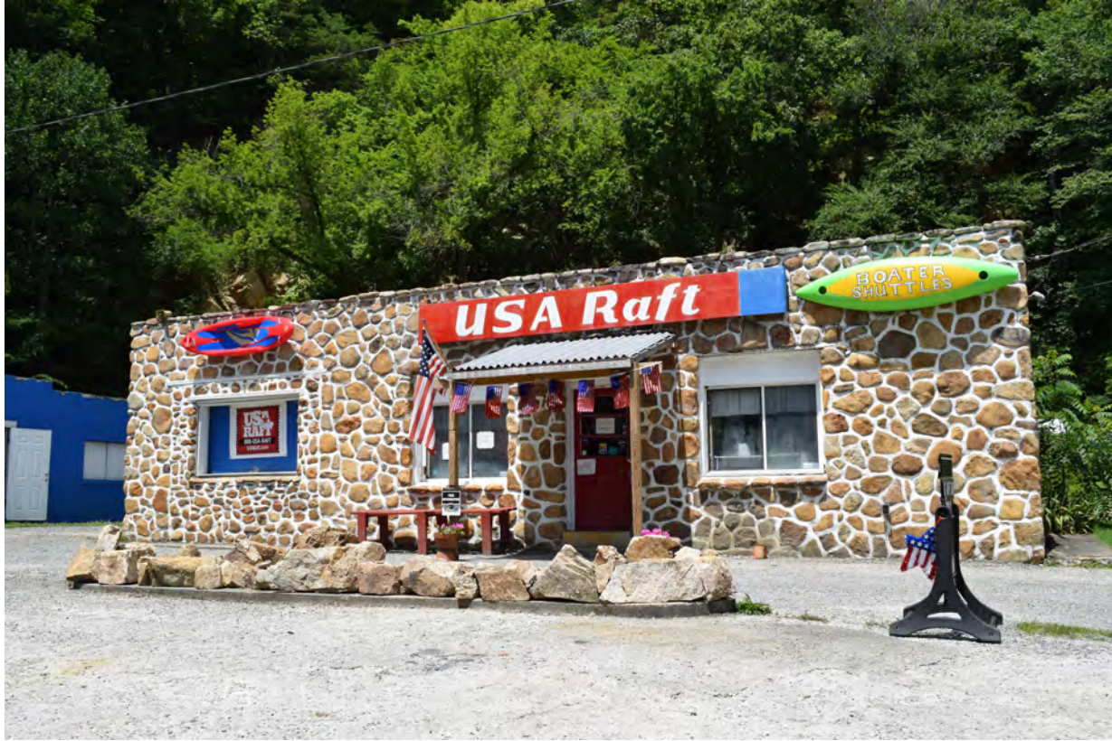
Store at 13490 US 70 near Marshall, view to the northeast
