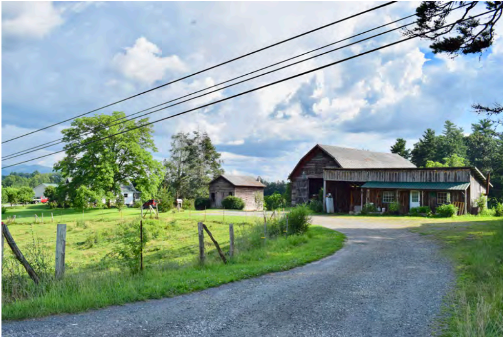
Outbuildings on the Robinson Farm, view to the southwest
