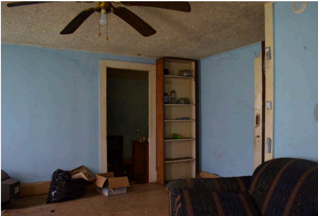
First floor parlor, view to the northeast
