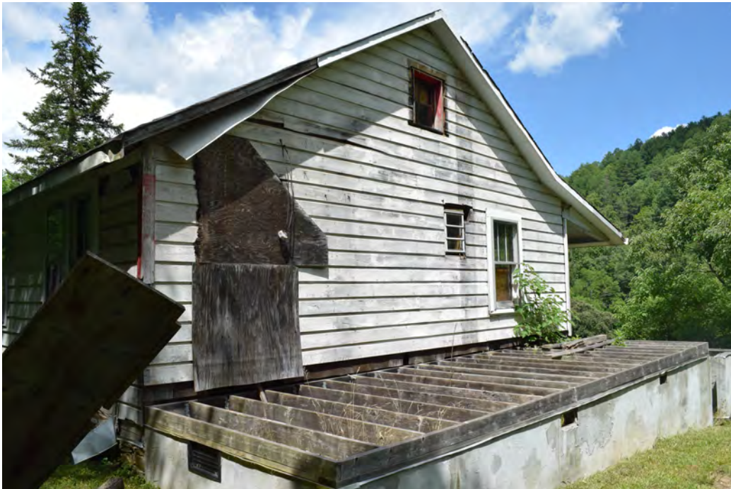
West gable end of house, view to the southeast
